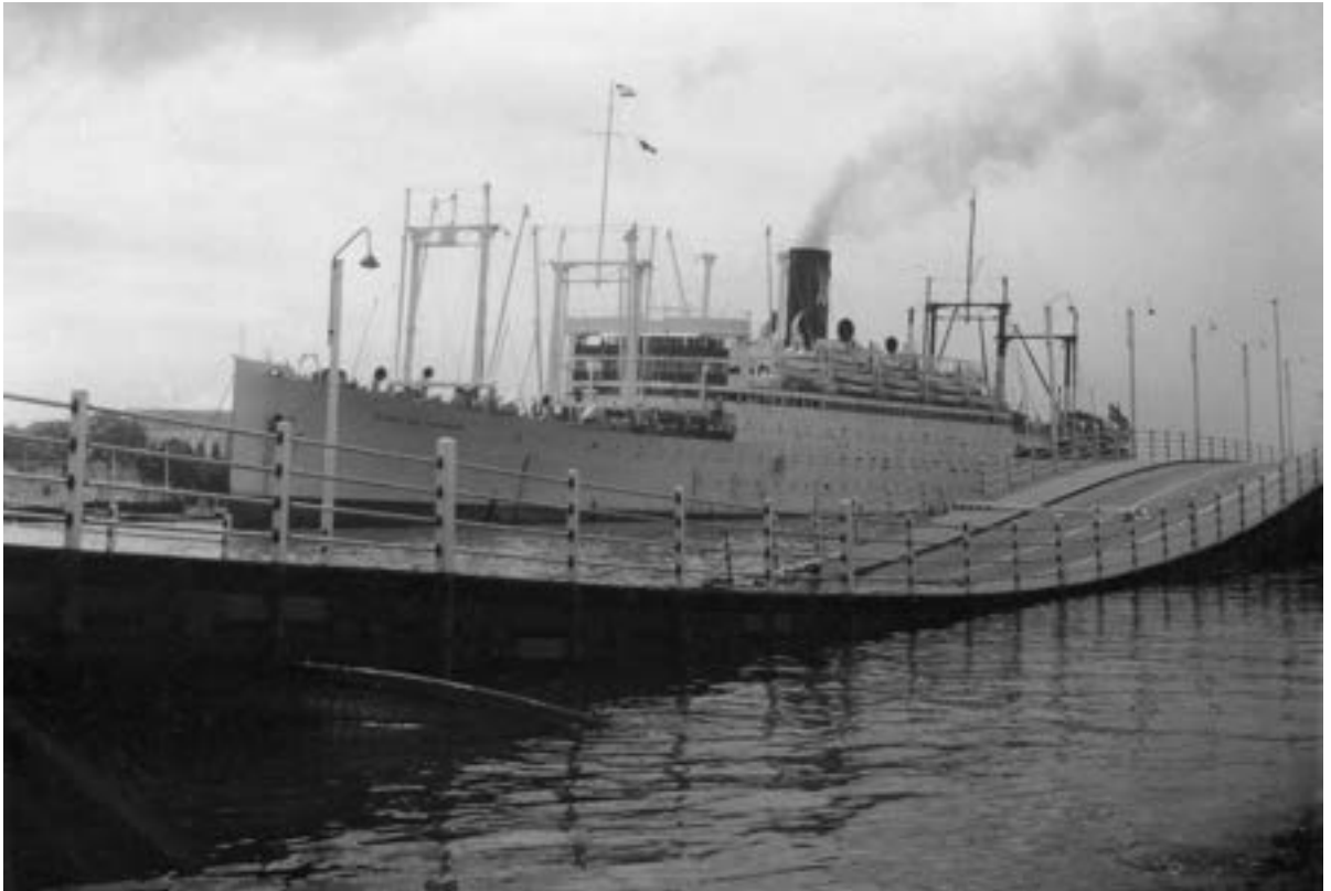
It was in February of that post-war year that the same Cabo de Hornos vessel collided into the Queen Emma Bridge spanning Curaçao's port. Collection Benjamin Gomes Casseres-06-84-0895
